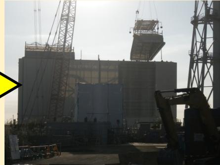
Reactor 1 was furnished with a cover in order to reduce the amount of radioactive substances being released in October, 2011. Currently the cover is being dismantled in preparation for the removal of rubble (October, 2015)
