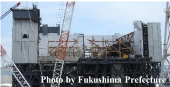
Installing a large cover for Unit 1
