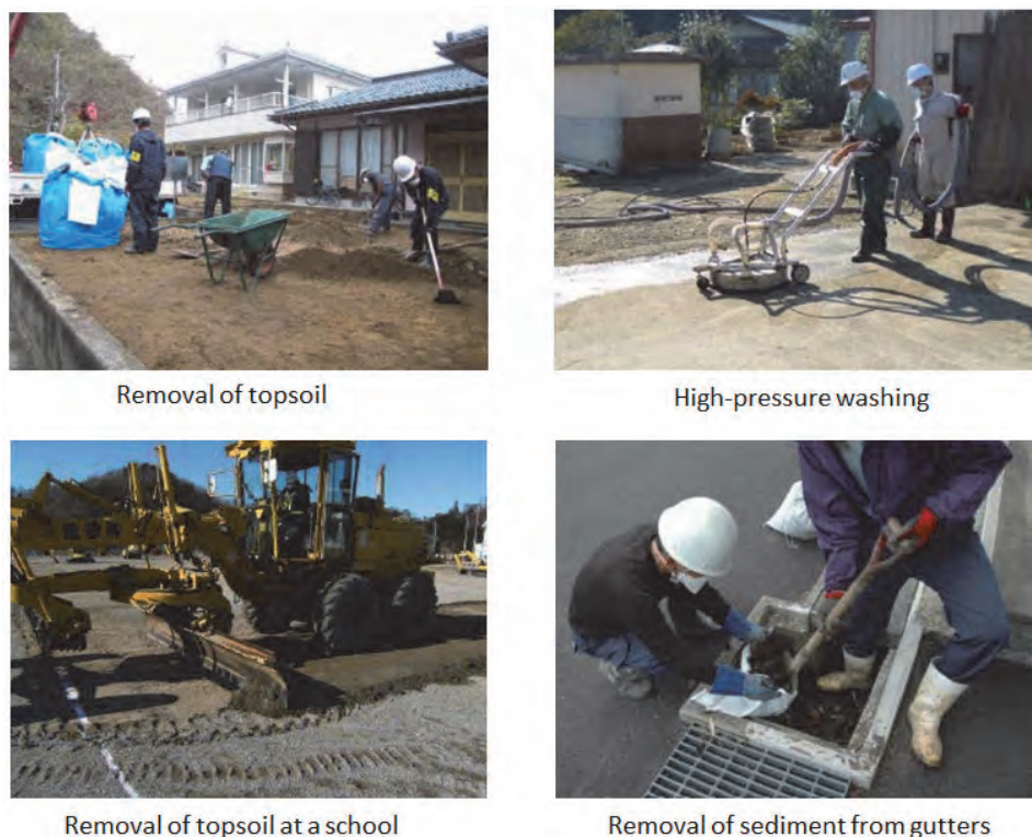
FIG. 5.8. Main decontamination techniques (Photo credit: Fukushima Prefecture)
